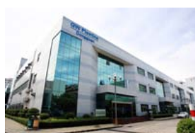
The An-Li High Tech Park in Dongguan is home to GW Plastics' China operation.
